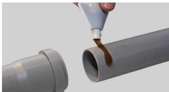
When inserting, the ring seal must be free of lubricant. Center up the spigot end of the pipe and push until the pipe end reaches the end of the socket.
